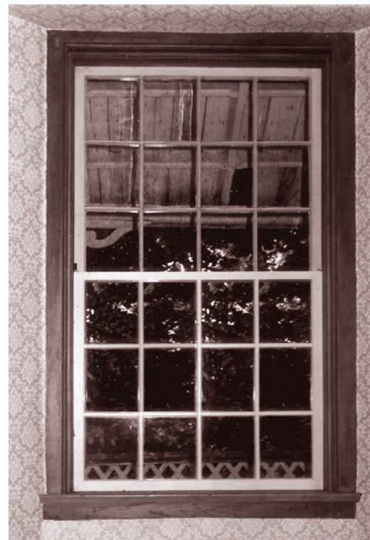
This would be described as a 12 over 12 window sash (Photo: Su Murdoch)
