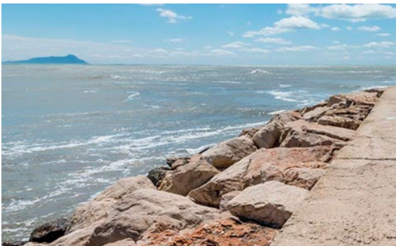
Rock toe protection for existing seawall.
