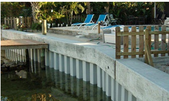
Concrete cap on steel sheet pile wall.
