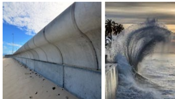
Recurved parapet wall added to seawall.
