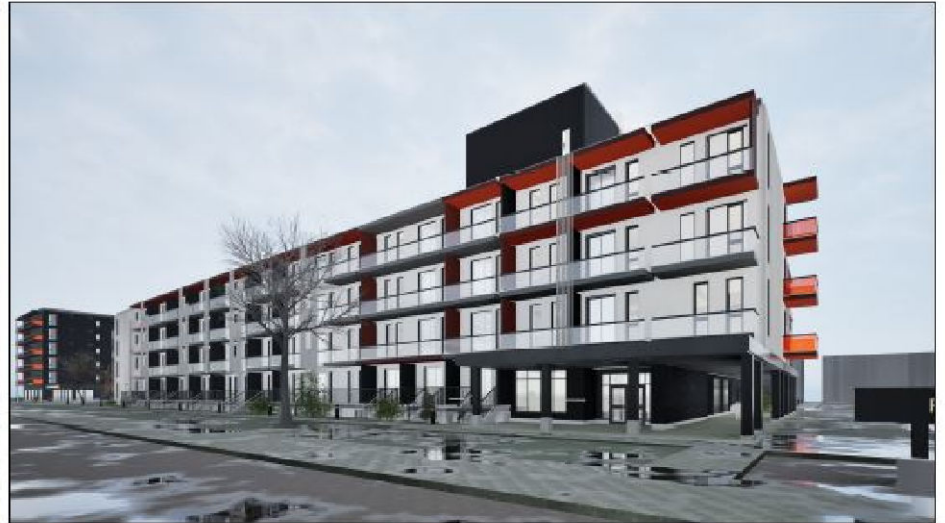
COURTYARD LOOKING ON NORTH BUILDING
