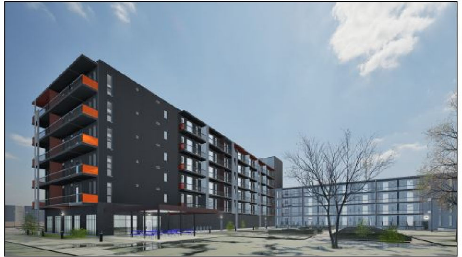
SOUTH EAST SIDE OF SOUTH BUILDING
